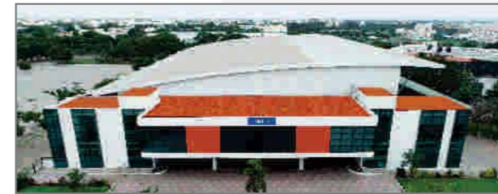
Exhibition Area : 5000 sq.m (53,800 sq.ft) 100m x 50m Minimum Roof Height 9 mts Exhibit Vehicle Entrance : 4.6m width x 5m height Heavy-duty flooring
